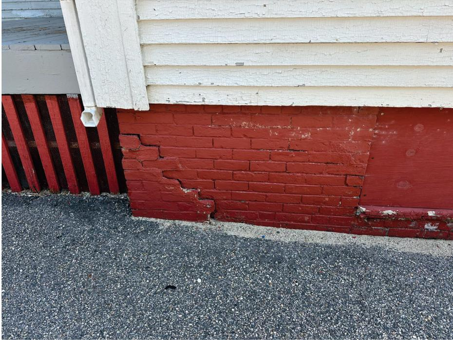
Brick displacement along Southeast perimeter wall
