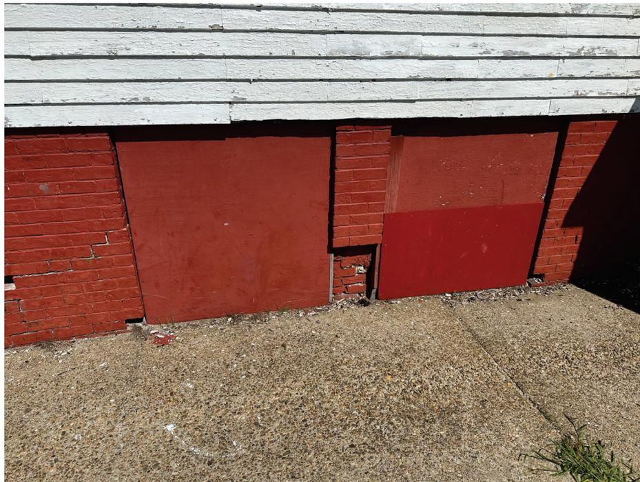
Missing brick and brick displacement along Southeast perimeter wall
